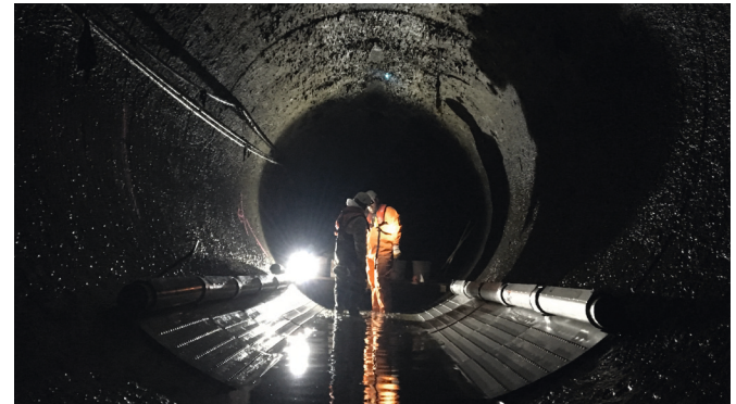
Heat exchangers in the sewage
