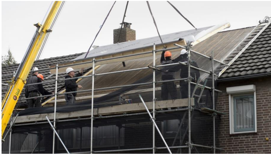
Figure 10: Placing of solar panels onto houses of Woonbedrijf in Eckart Vaartbroek
