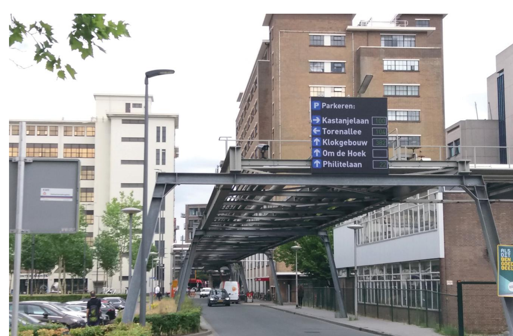
Dynamic parking management signpost at Strijp-S Credits: VolkerWessels
