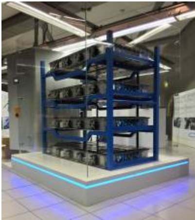
Figure 20: The second-life battery storage at BMW, Leipzig 32
